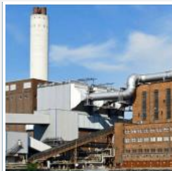
Relocation Feasibility Study on 119MW Hastedt Power Station Coal Fired Thermal Power Plant. • Siemens S.T. • Heidelergen S.G.
