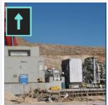
Relocation Feasibility Study on 180MW Workington Natural Gas Fired Combined Cycle Power Plant. • GE LM6000 PG G.T. • Skoda Condensing S.T. • Skoda HRSG
