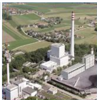
Relocation Feasibility Study on 165MW Riederschbach Coal Fired Thermal Power Plant. • Westinghouse S.T. • F. Tosi S.G.
