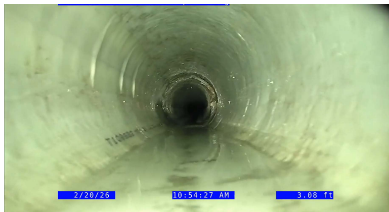
Most of the old 6-inch and 8-inch pipe was relined with cured in place plastic pipe.
