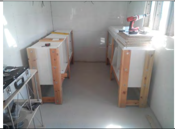
Benches Being Installed
