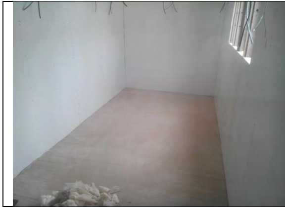
Garage Lining Completed
