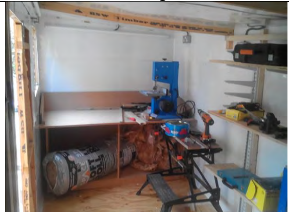
Further Internal Construction
