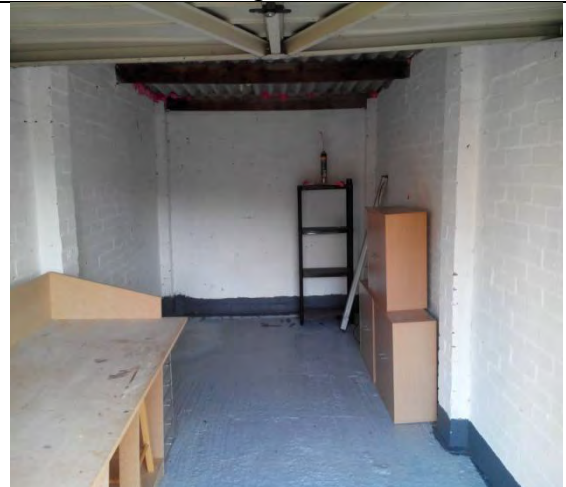
Concrete Floor in Garage
