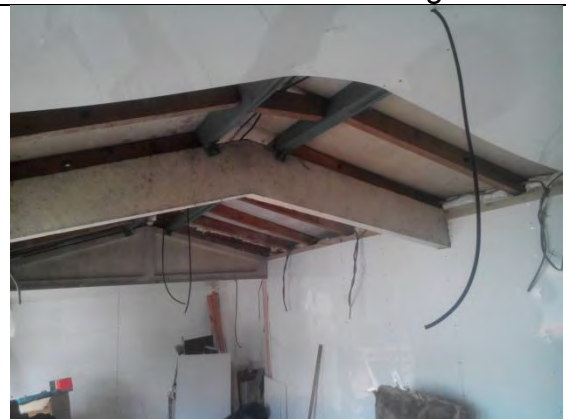
Lining and Wiring the Garage
