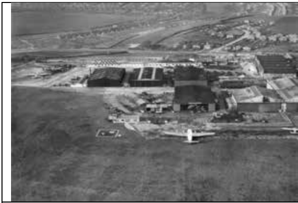
Photo 05 Percival Works Luton
