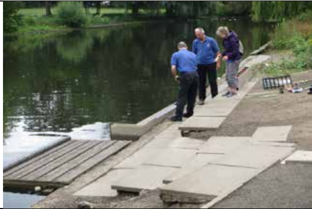
Harbour Being Assembled
