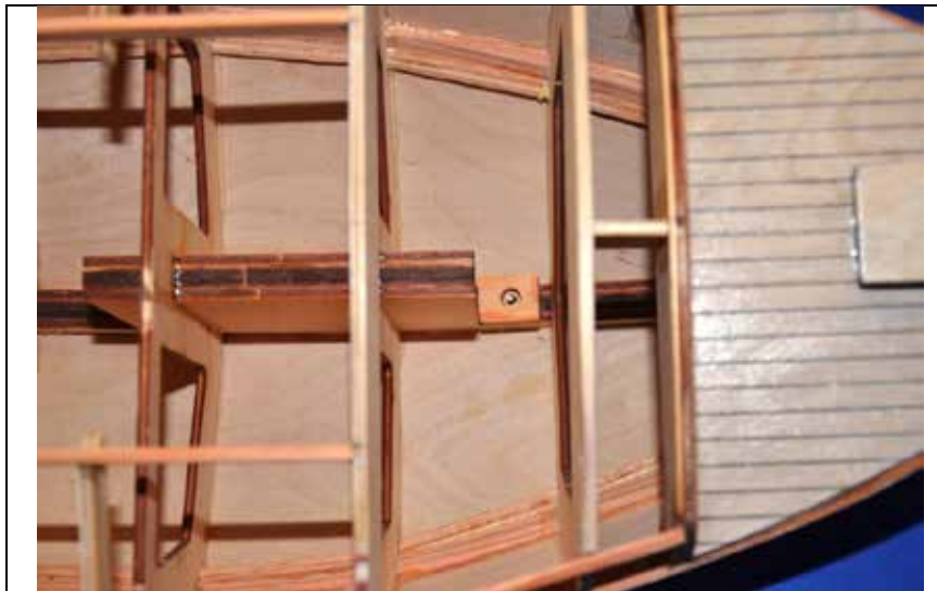
Photo 14. Mast Footing Bonded into Position
