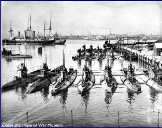
'A', 'B', and 'C' class submarines alongside Fort Blockhouse, Gosport, the Submarine Service Headquarters, circa 1910.
