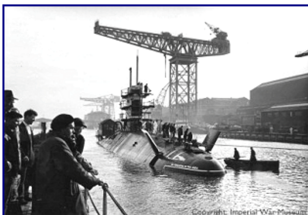
Dreadnought during fitting out at Barrow-in-Furness, November 1962.
