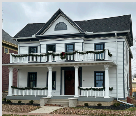
115 Frost Parkway AFTER
