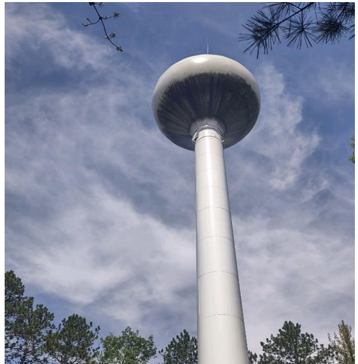
VCARC Repeater antenna is shown at the top.
