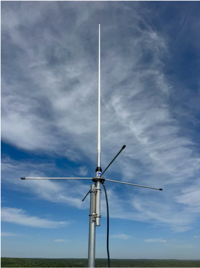
New Hustler G6-270R antenna mounted in place
