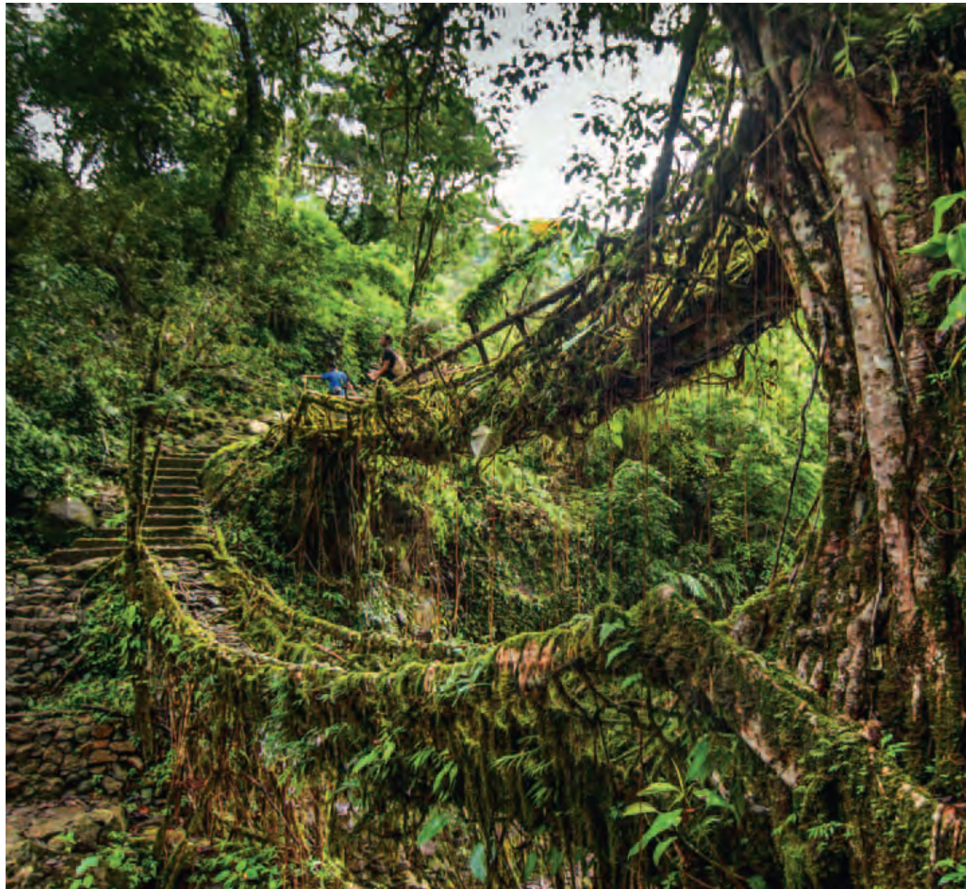
The residents of Nongriat have started growing a third level to their famous double-decker bridge in an effort to retain the village's claim to fame.
