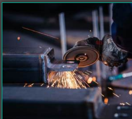
STEEL FABRICATION WORKS
